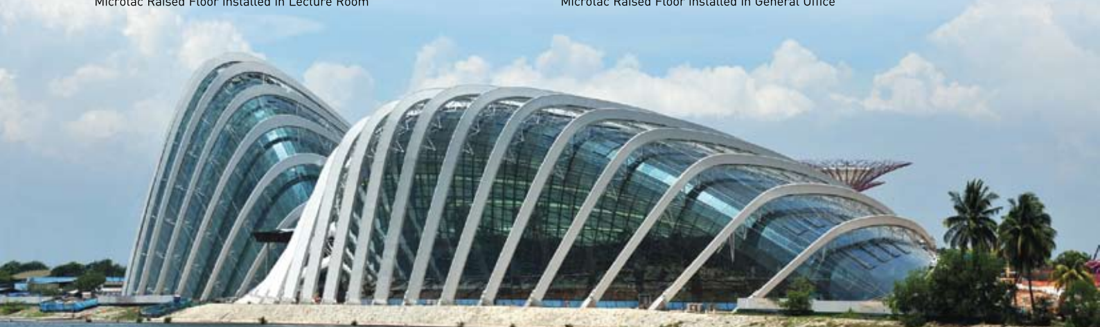
Garden by the bay (Microtac Raised Floor System)
