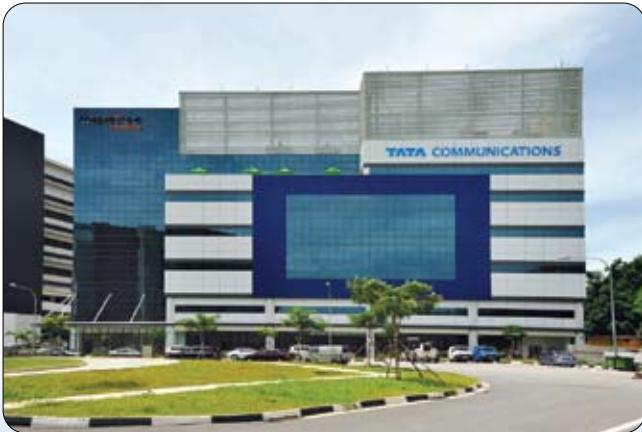
TATA Communications (Microtac Raised Floor System)
