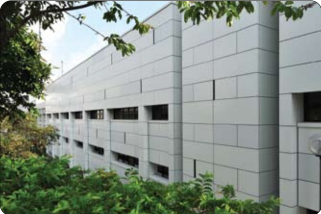
NUH [External Wall Cladding]
