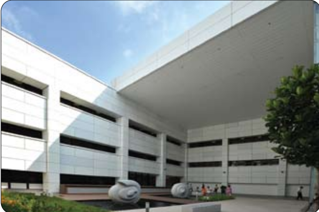
NUH [External Wall Cladding]
