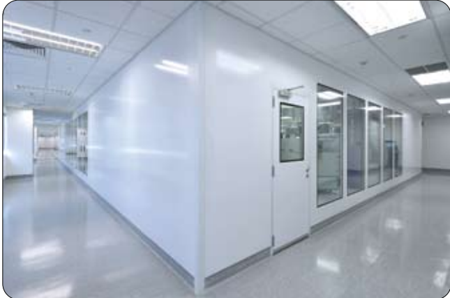
Medtronic Singapore Operations Pte Ltd (Aluminum Honeycomb Panel)
